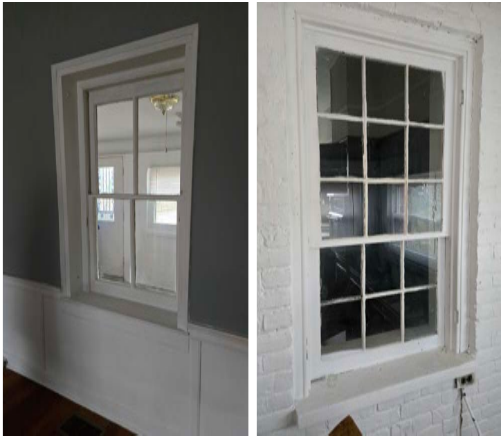
Historic interior windows from additions
