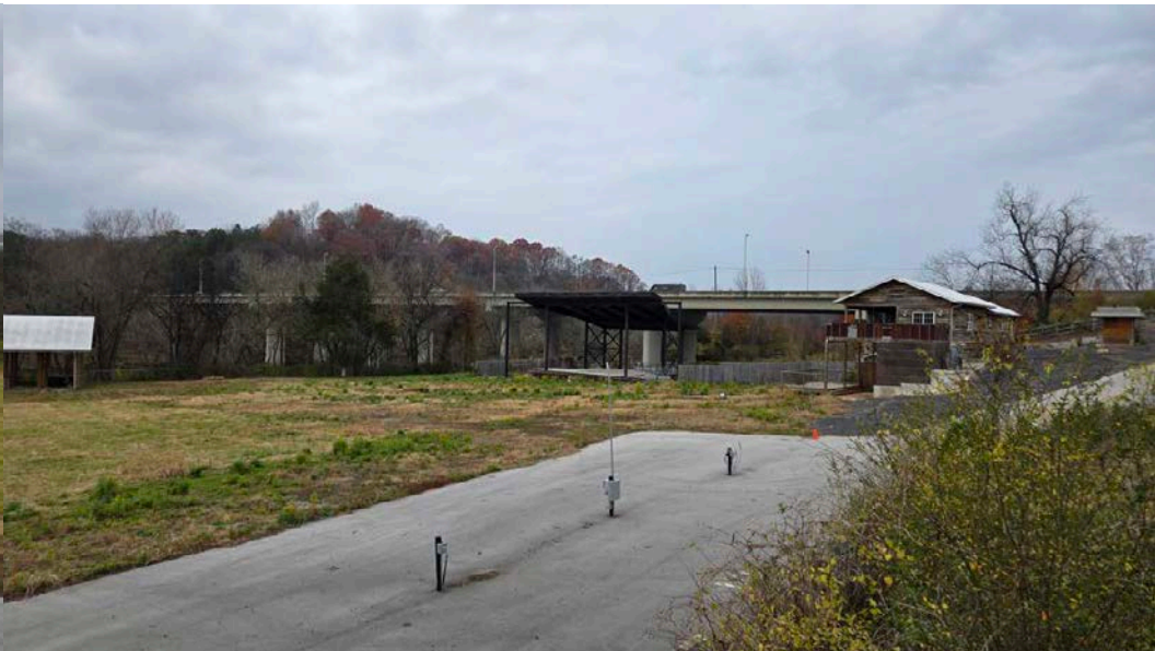
Existing site features of River Breeze Event Center
