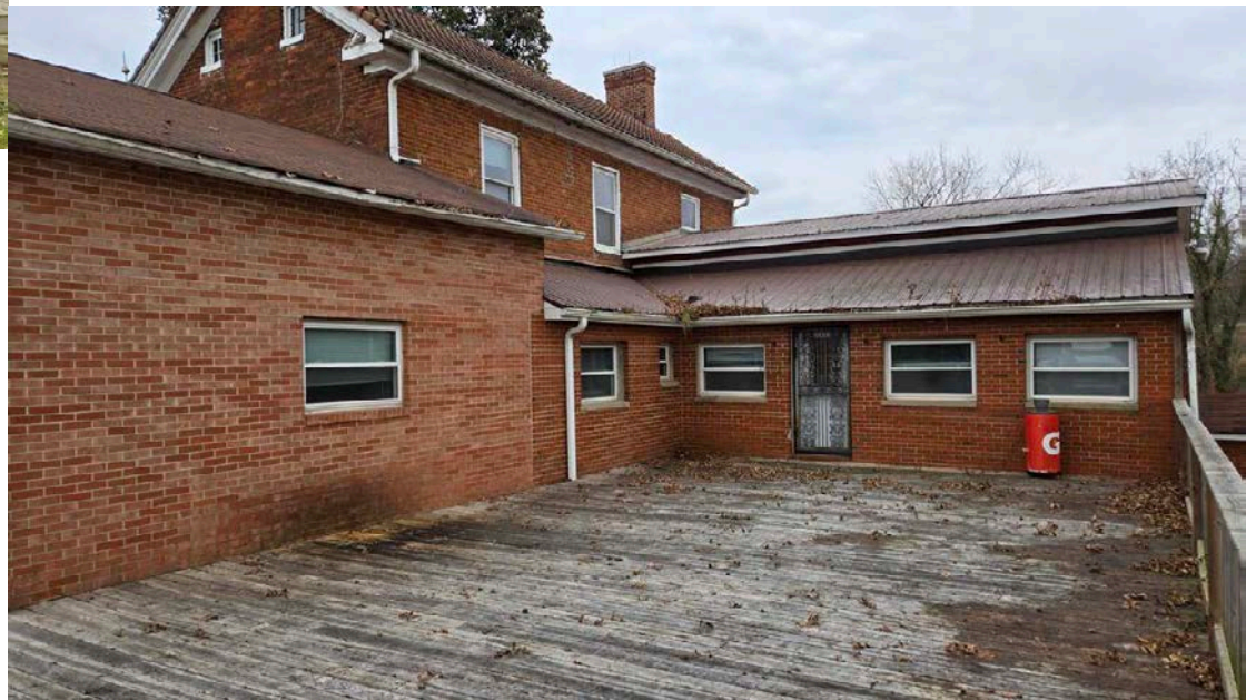
Rear elevation: 20 th century addition on interior of rear ell, rear view of side wing addition, wood shingles visible near partial cornice return, original gable window
