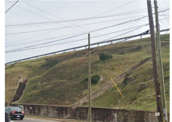
1. Existing Concrete Stairs along Sevier Ave.
