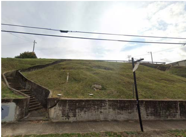
2. Existing Concrete Stairs along Sevier Ave.
