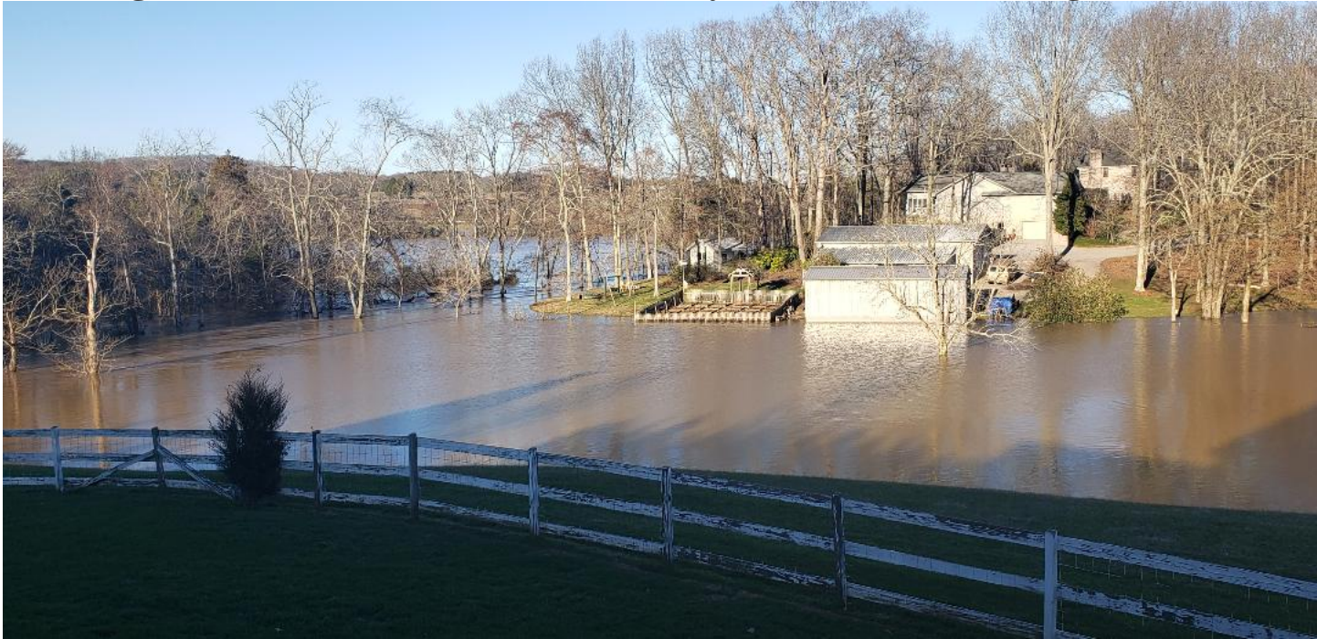
#10 Diagonal Backside of 8520 West Emory Road (After flooding)
