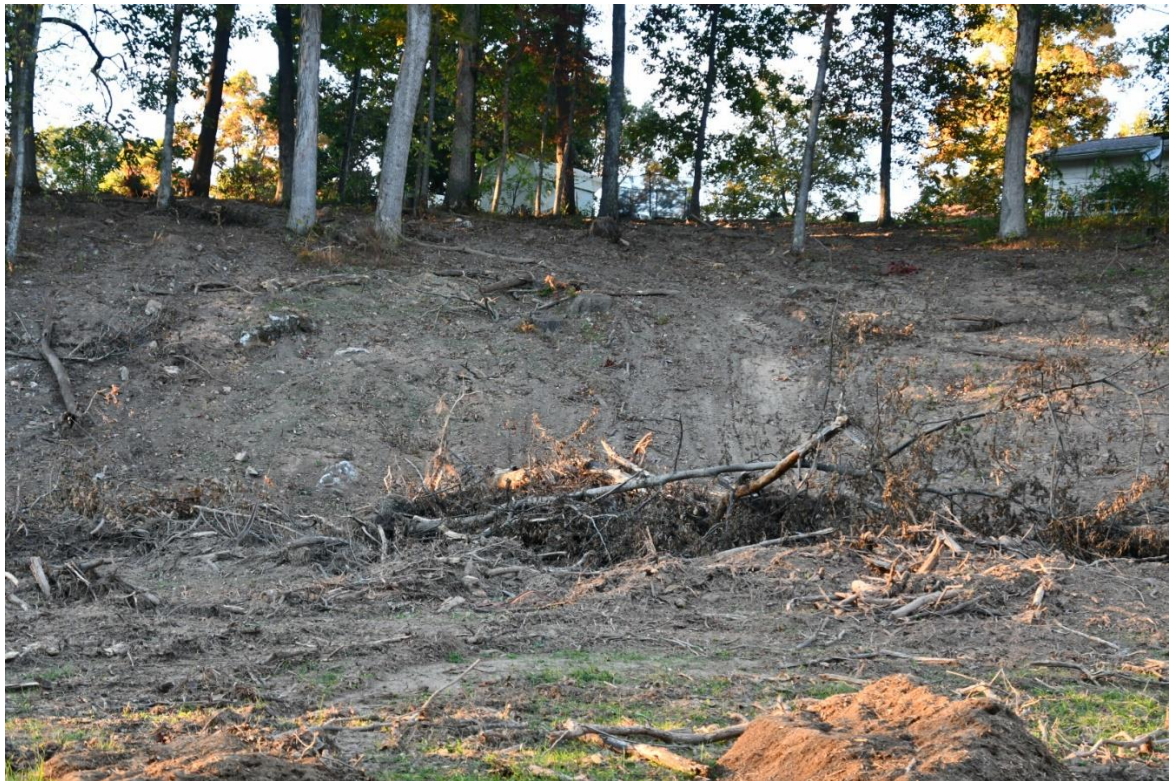
Hill sides stripped of 90% of the trees creek at base of hill is filled in.....Zero erosion control....danger!
