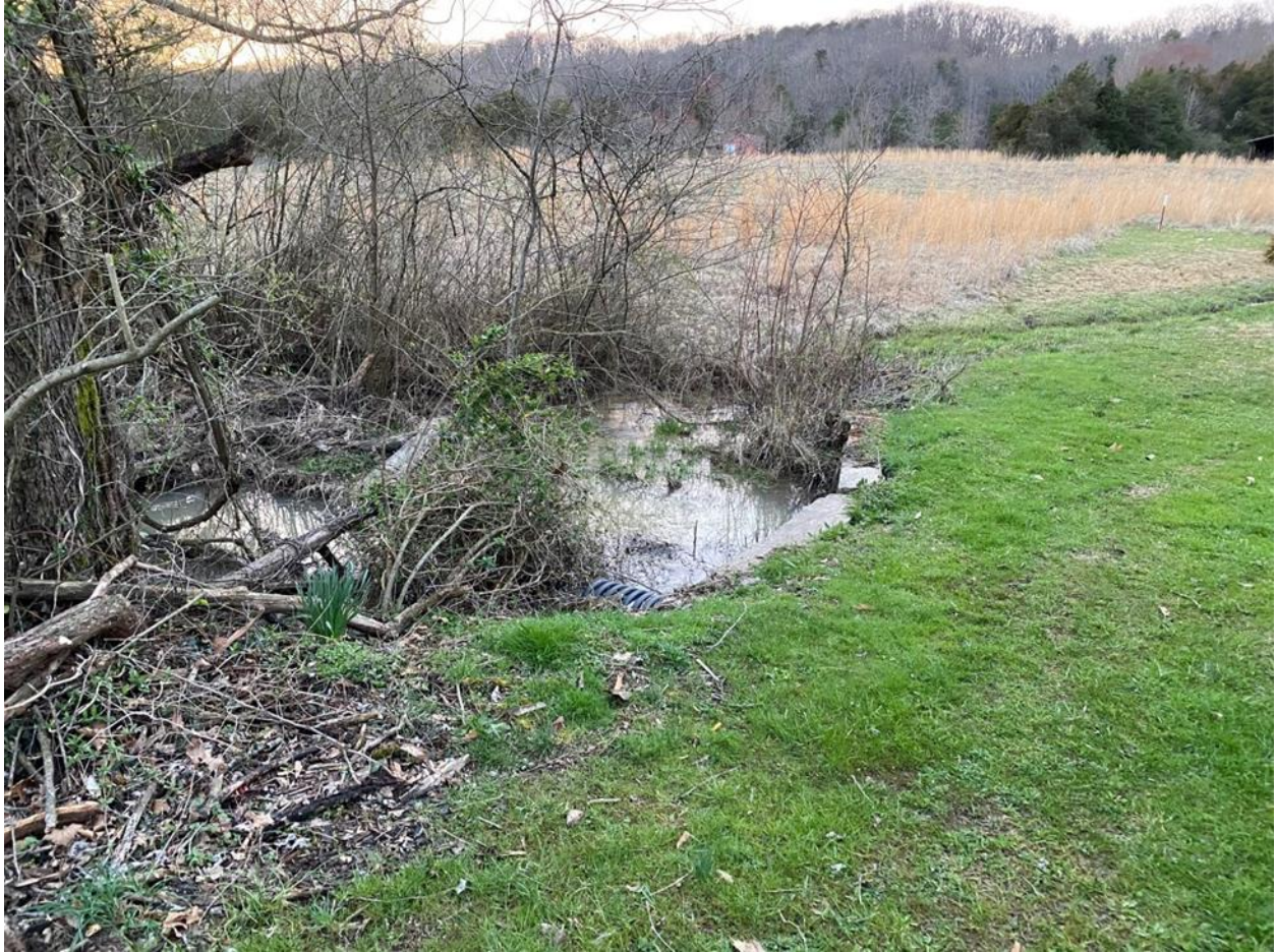
Figure 3 - Water backed up from damage to the blue line stream.
