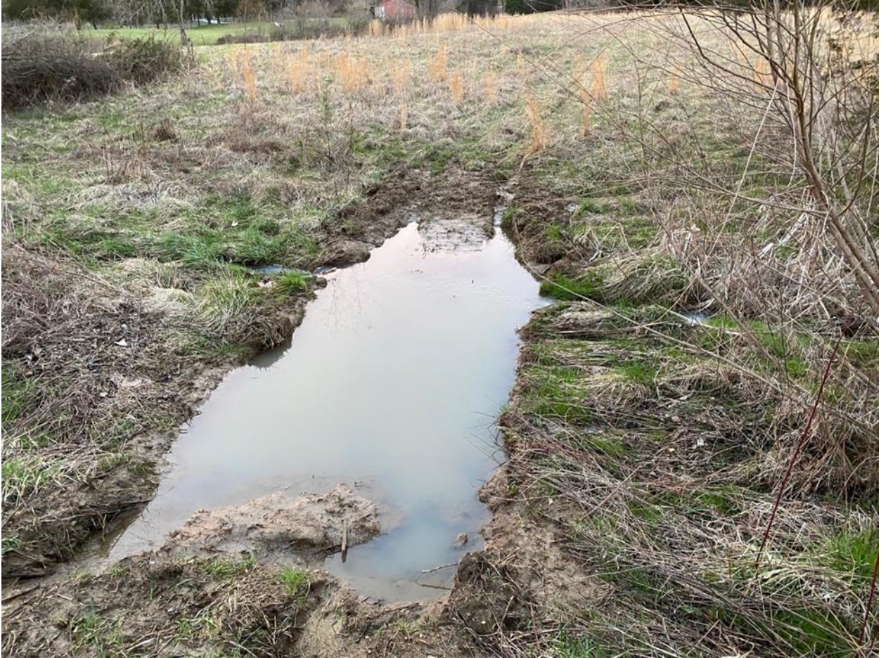
Figure 2 - Drilling machine caused damage to blue line stream causing water to back up on our property during rain events.
