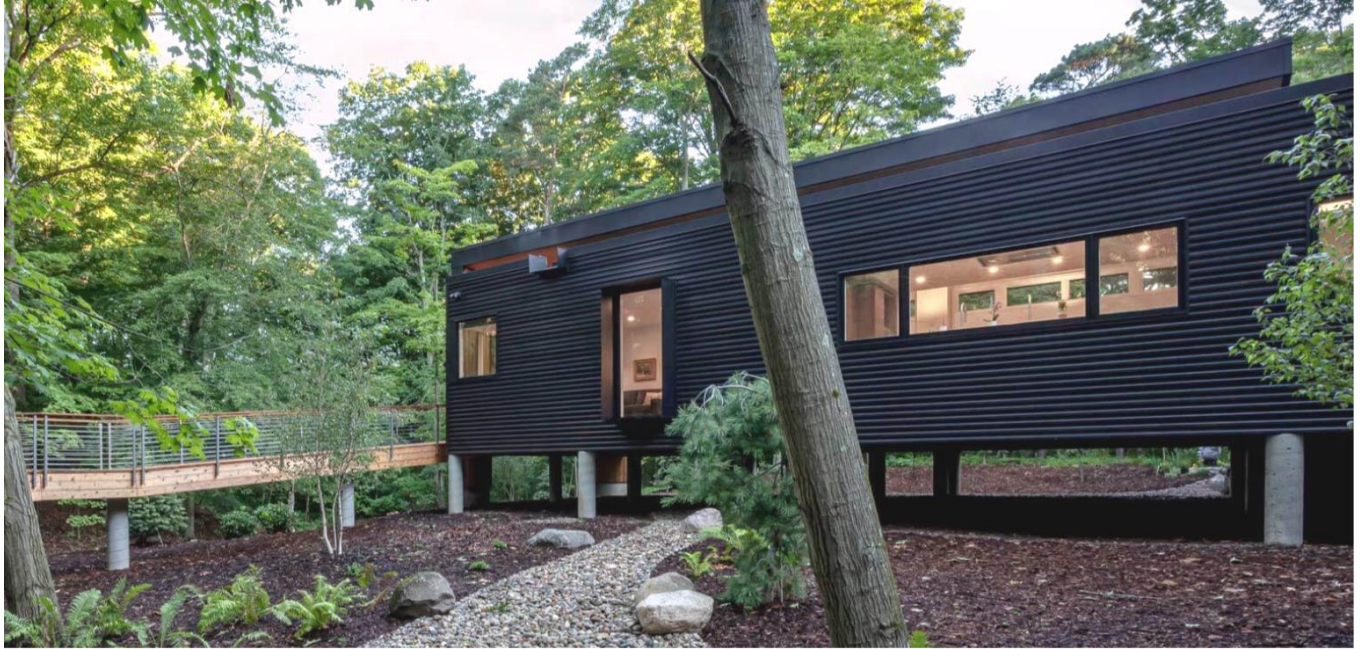
Piers allow for natural drainage Notice minimal site grading and preservation of existing vegetation
