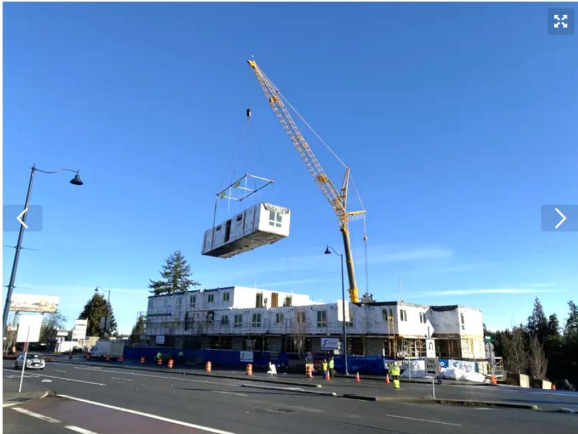
1 of 2 | A multistory residential apartment building is shown being set on a podium manufactured by NRB Modular Solutions for Synergy Inc. (Courtesy of NRB Modular Solutions)
