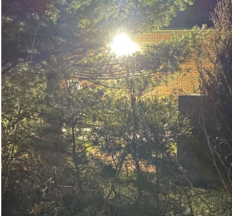
Figure 7 - Rear of 5904 Washington Pike from rear property line. Glare from wall pack. Measured 0.22 footcandles vertical illuminance. March 14, 2022
