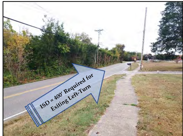
View of Sight Distance on Tipton Station Road at the Proposed Entrance Location (Looking Northeast)
