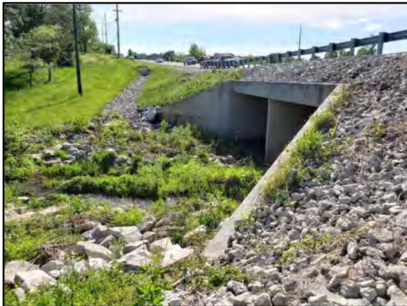
Box Culvert for Kerns Branch on East Emory Road (Looking West)
