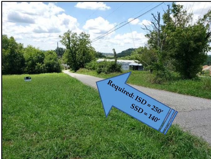
View of Sight Distance on Number Two Drive at Proposed Road "A" (Looking South)
