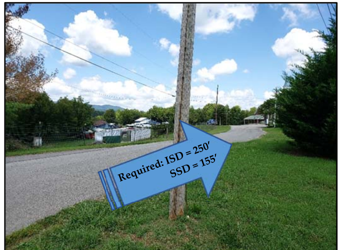
View of Sight Distance on Number Two Drive at Proposed Road "A" (Looking North)
