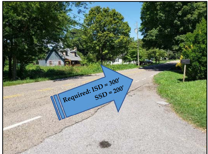
View of Sight Distance on Mascot Road at Number Two Drive (Looking East)
