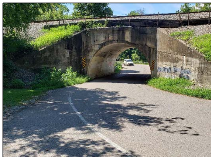
View of Mascot Road at NS Railroad Underpass (Looking North)
