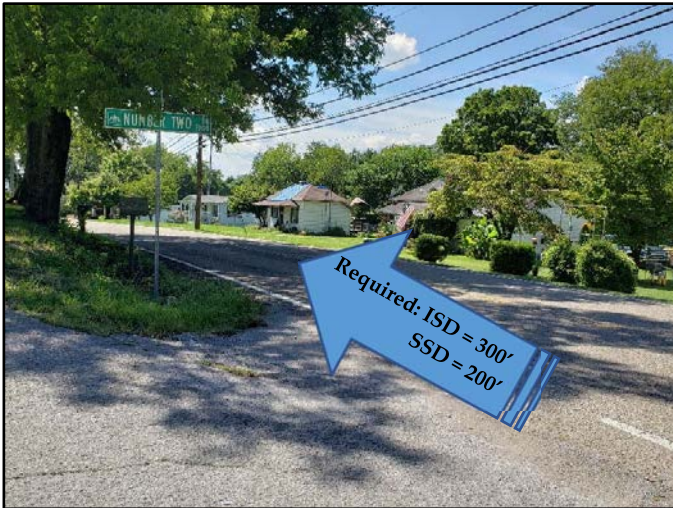
View of Sight Distance on Mascot Road at Number Two Drive (Looking West)
