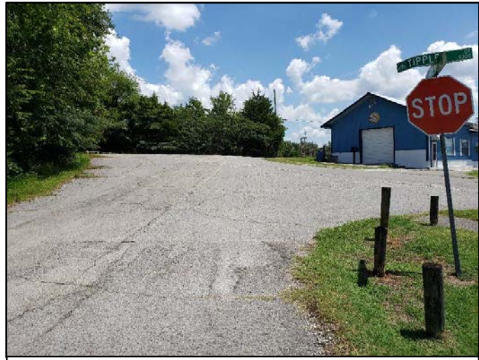
View of Number Two Drive Approach at Tipple Drive (Looking Southeast)
