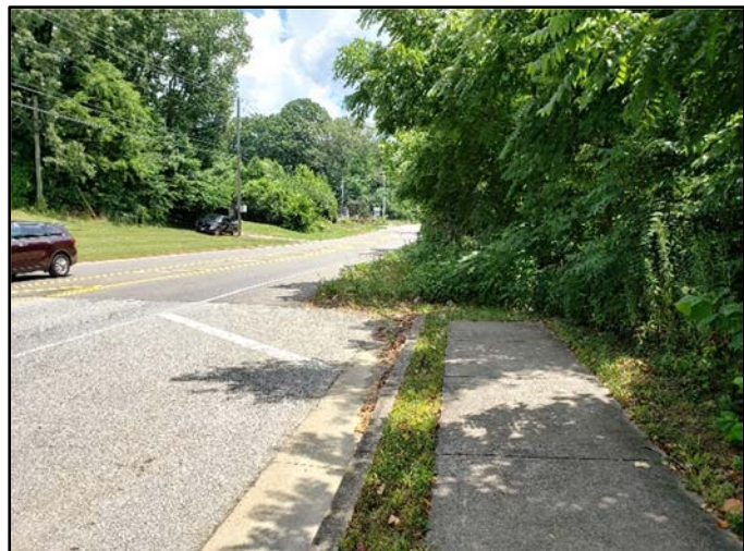
End of Sidewalk on West Side of Dry Gap Pike (Looking South)
