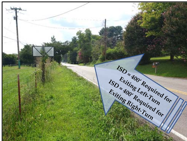
View of Sight Distance on Millertown Pike at the Proposed Entrance Location (Looking Southwest)
