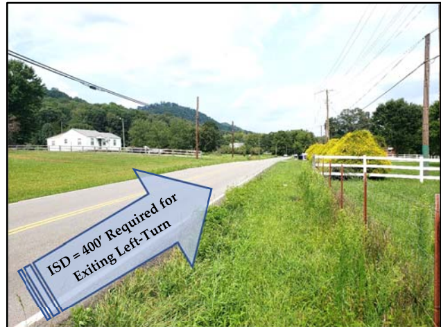
View of Sight Distance on Millertown Pike at the Proposed Entrance Location (Looking Northeast)
