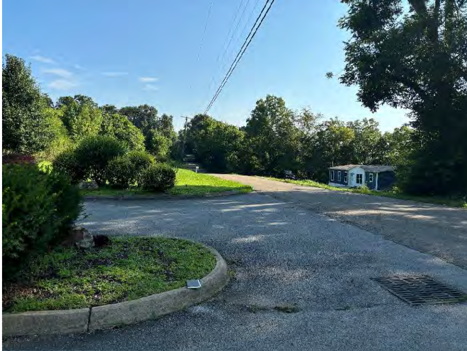
Maloneyville Road at Whisper Ridge Lane – Looking Left (Northbound)
