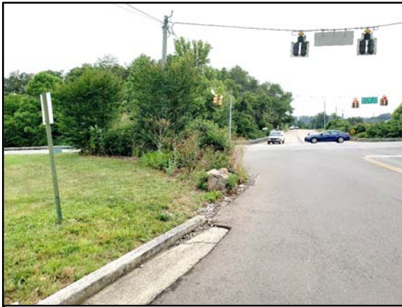
Reduced Sight Distance at Southwest Corner of Intersection of West Governor John Sevier Highway at Mountain Grove Drive / West Norton Road due to Uncontrolled Vegetation
