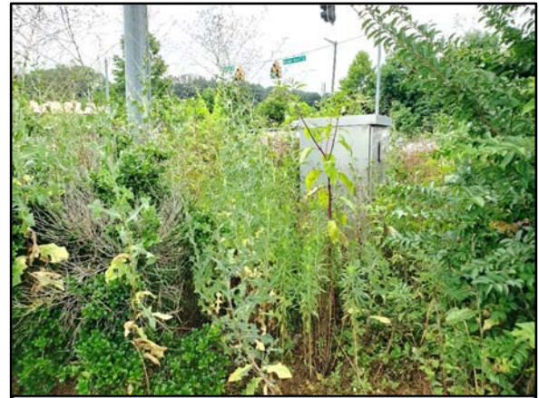
Traffic Signal Cabinet Surrounded by Uncontrolled Vegetation at Southwest Corner of Intersection of West Governor John Sevier Highway at Mountain Grove Drive / West Norton Road
