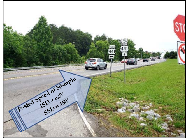
View of Sight Distance on West Governor John Sevier Highway at Proposed East Entrance at the Weigel's Driveway (Looking East)
