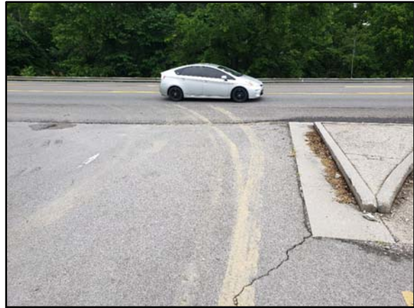
Mud Tracks on Entering Lane from Motorists Illegally Turning Left onto West Governor John Sevier Highway from the Weigel's Driveway Approach
