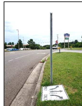
Damaged Traffic Road Sign on Mountain Grove Drive
