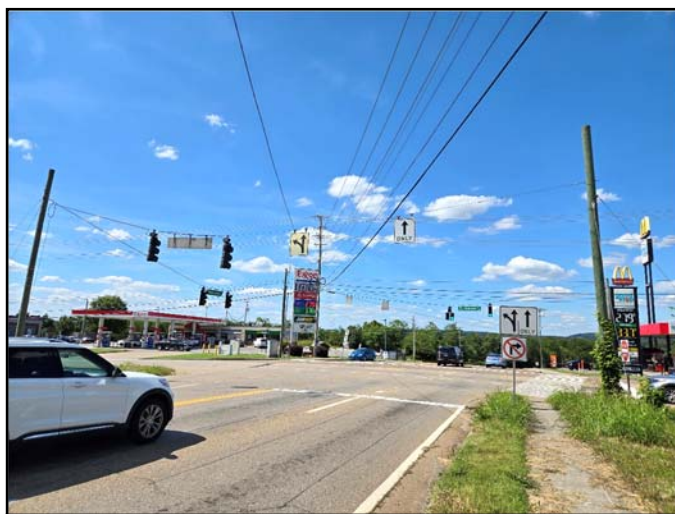
Lane Use Control Signs on Walker Springs Road Northbound Approach at Walbrook Drive
