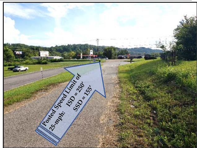
View of Sight Distance on Jim Jones Lane at Road "A" Proposed Entrance (Looking South)
