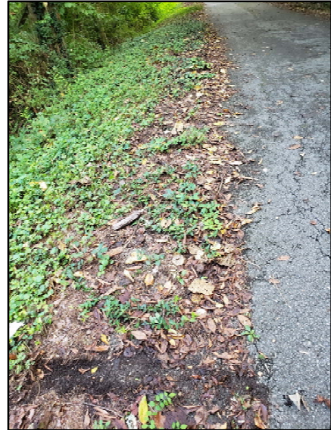
Existing Jim Jones Lane Pavement and Edge Obscured due to Organic Debris
