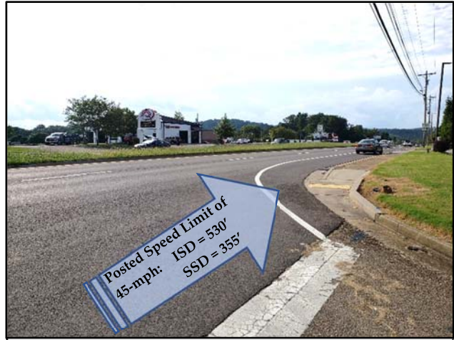
View of Sight Distance on Oak Ridge Highway at Jim Jones Lane (Looking West)
