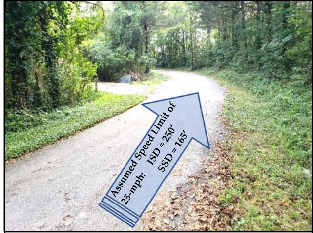
View of Sight Distance on Jim Jones Lane at Road "B" Proposed Entrance (Looking South)
