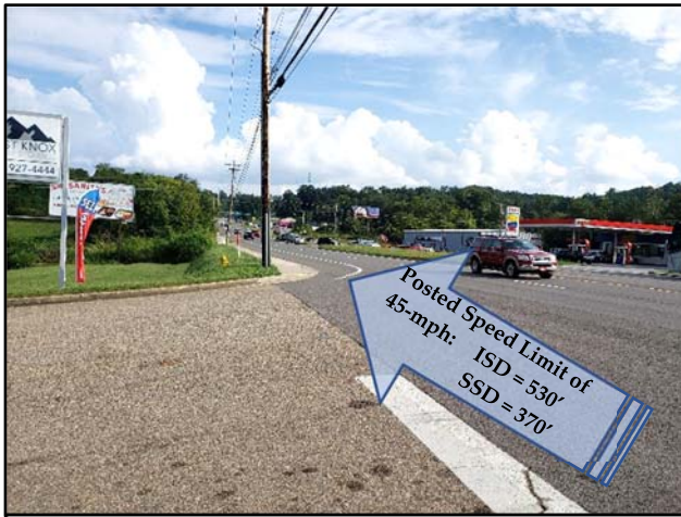
View of Sight Distance on Oak Ridge Highway at Jim Jones Lane (Looking East)
