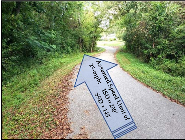
View of Sight Distance on Jim Jones Lane at Road "B" Proposed Entrance (Looking North)
