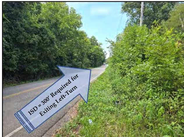
View of Sight Distance on Harvey Road at the Proposed West Entrance Location (Looking North)
