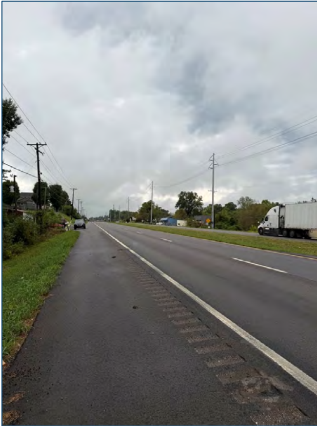
Looking left along Andrew Johnson Highway (US 11E) from the proposed site access. Approx. Sight Distance: 950 ft
