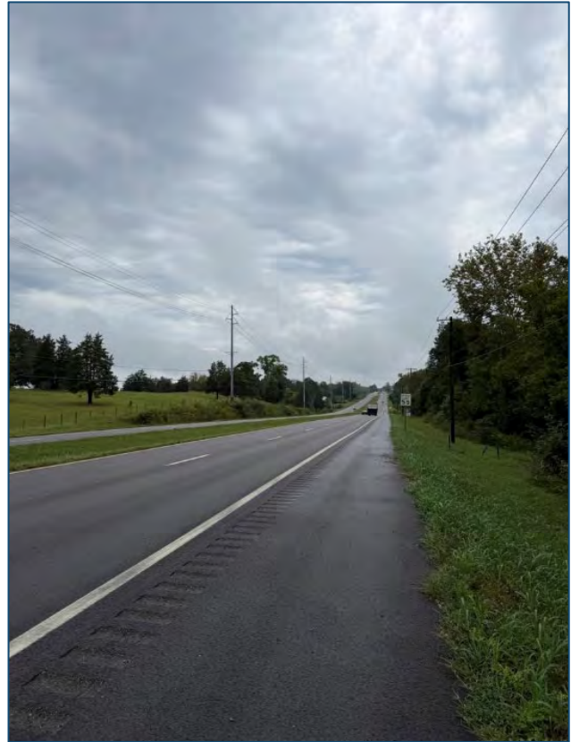
Looking right along Andrew Johnson Highway (US 11E) from the proposed site access. Approx. Sight Distance: 1,000+ ft
