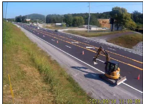
Image of Lane Closure during Traffic Count
