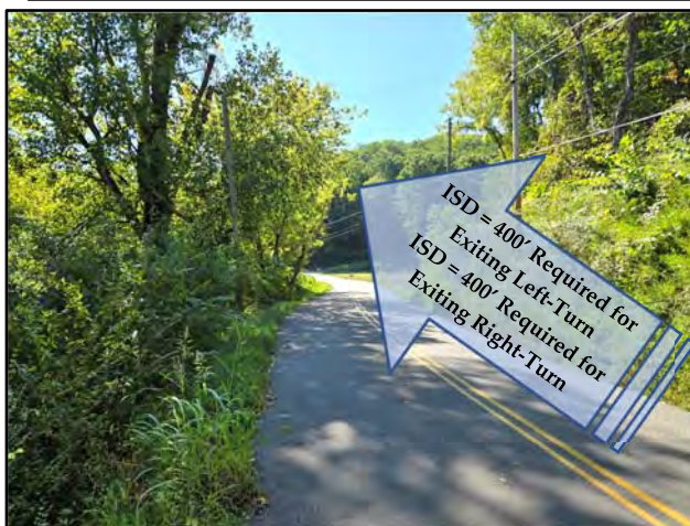
View of Sight Distance on Pickens Gap Road at the Proposed Entrance (Looking South)
