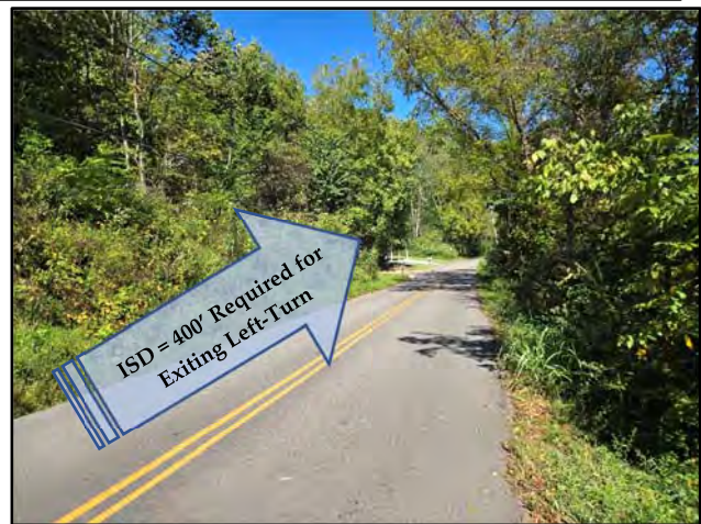
View of Sight Distance on Pickens Gap Road at the Proposed Entrance (Looking North)
