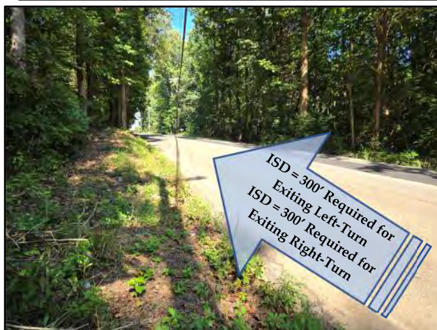
View of Sight Distance on George Williams Road at Proposed Entrance Location (Looking East)
