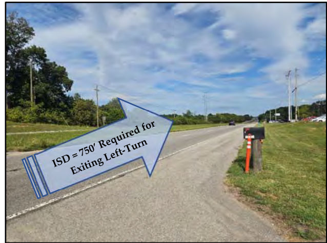
View of Sight Distance on Asheville Highway at the Proposed Entrance (Looking East)
