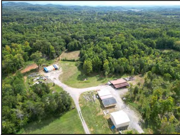
Existing Structures on Proposed Development Property (Looking South)
