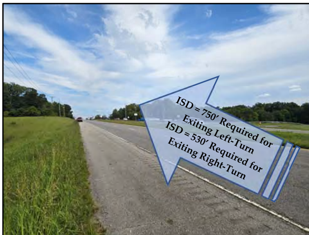
View of Sight Distance on Asheville Highway at the Proposed Entrance (Looking East)
