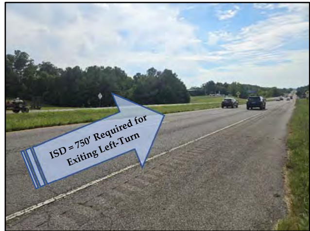
View of Sight Distance on Asheville Highway at the Proposed Entrance (Looking West)
