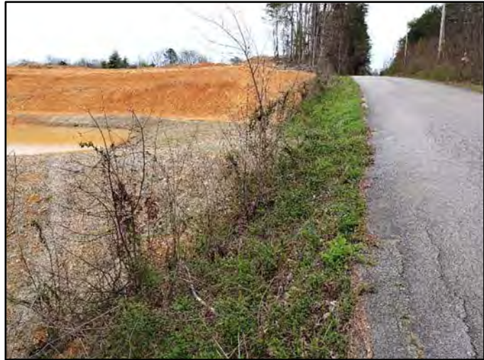
North Side of Hatmaker Lane Adjacent to Stormwater Detention Pond for Windsor Forest
