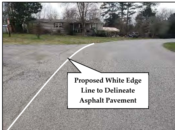
Large Expanse of Asphalt Pavement at 90° Horizontal Curve (Looking South)
