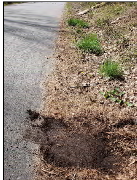
Road Pavement and Edge Obscured due to Organic Debris
