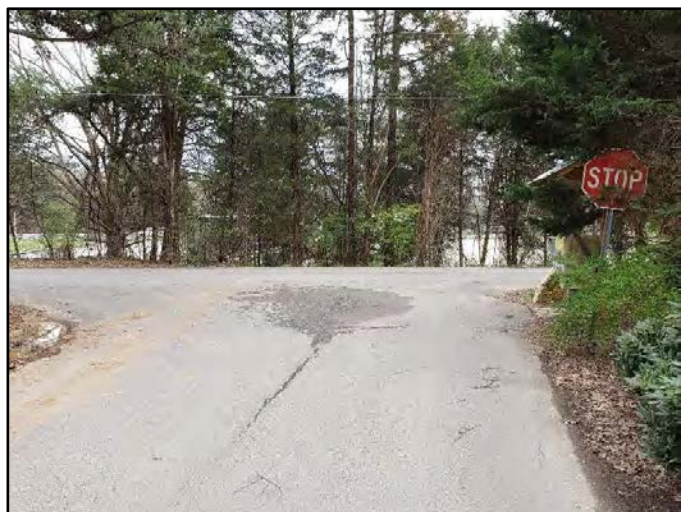
Stop Sign (R1-1) Obscured at Hopper Lane Approach at Hatmaker Lane
