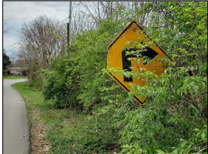
Turn Sign (W1-1R) Obscured and Damaged – Located Prior to 90° Horizontal Curve (Looking South)
