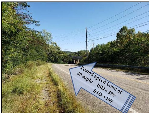
View of Sight Distance on Fox Road at the Proposed Entrance (Looking South)
