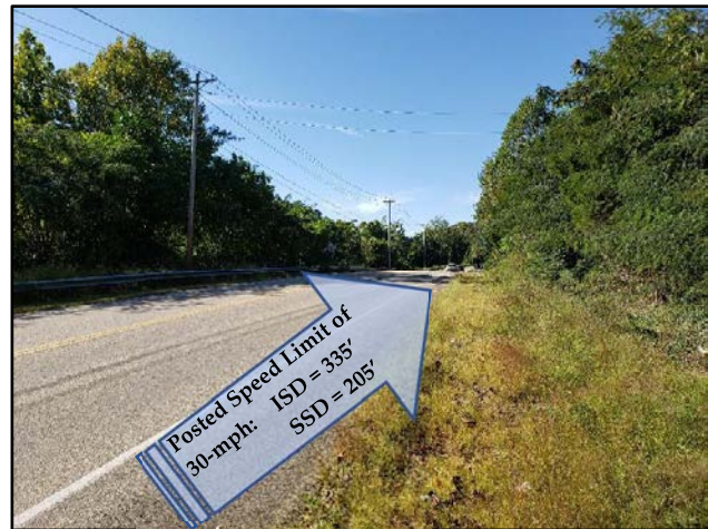
View of Sight Distance on Fox Road at the Proposed Entrance (Looking North)
