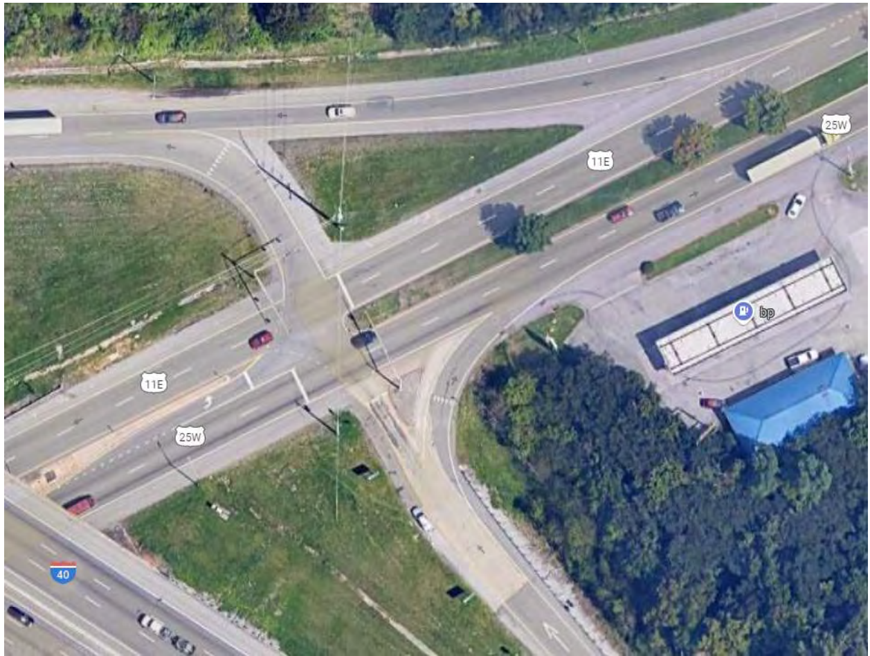
Asheville Highway at I-40 Westbound Ramp
