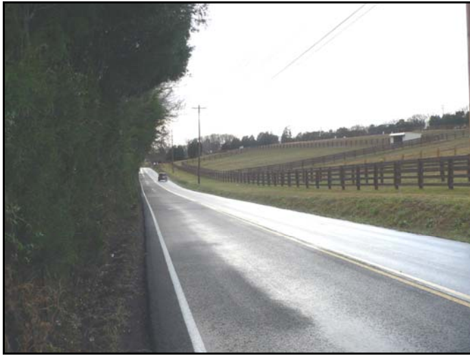
View of Hickory Creek Road from Proposed Roadway Tie-In (Looking Southwest)
