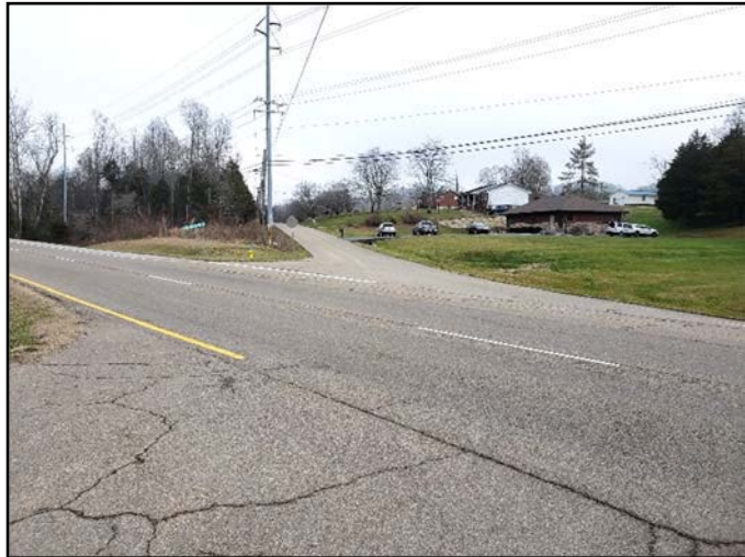
North Ruggles Ferry Pike (East Side) at Andrew Johnson Highway (Looking East)
