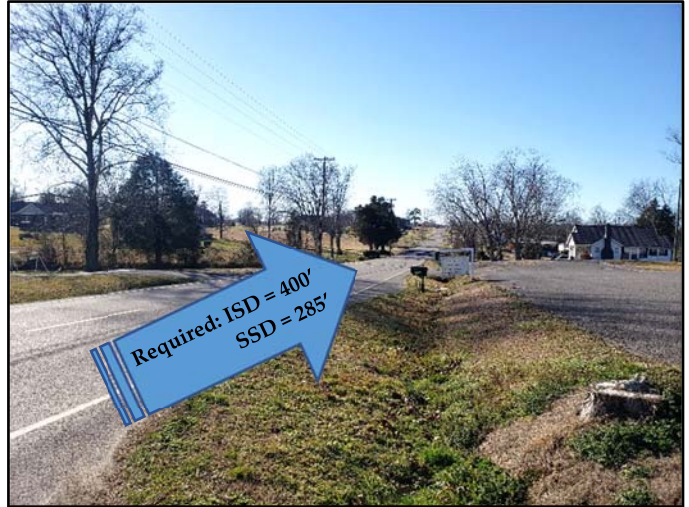
View of Sight Distance on North Ruggles Ferry Pike at Proposed Entrance - Blake Lane/Road "Q" Intersection (Looking West)
