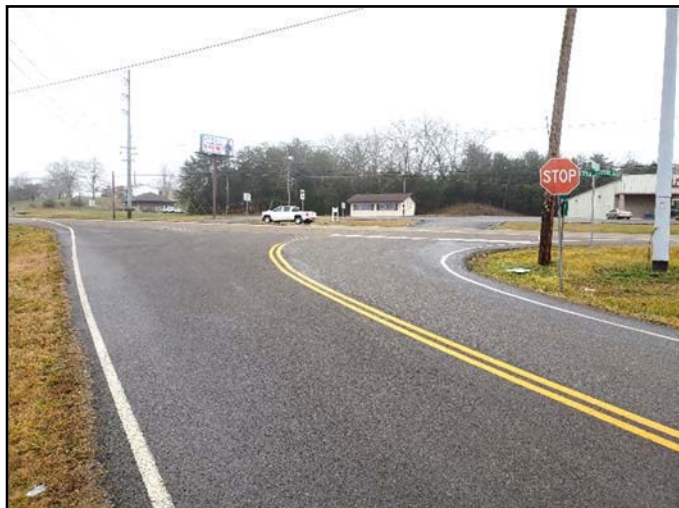
North Ruggles Ferry Pike (West Side) at Andrew Johnson Highway (Looking East)
