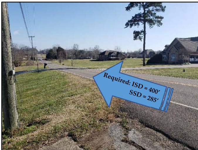
View of Sight Distance on North Ruggles Ferry Pike at Proposed Entrance - Road "A" Intersection (Looking East)
