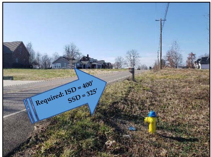
View of Sight Distance on North Ruggles Ferry Pike at Proposed Entrance - Road "A" Intersection (Looking West)
