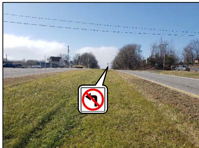
Median of Asheville Highway at North Ruggles Ferry Pike (Looking West)
