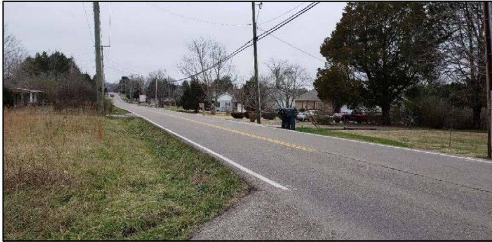
View of Sight Distance on East Emory Road (SR 131) Looking Southwest from Thomas Lane
