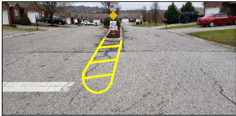
Proposed Yellow Pavement Markings in Front of Existing Raised Median on Rocky Mountain High Boulevard at East Beaver Creek Drive (Looking Northwest)
