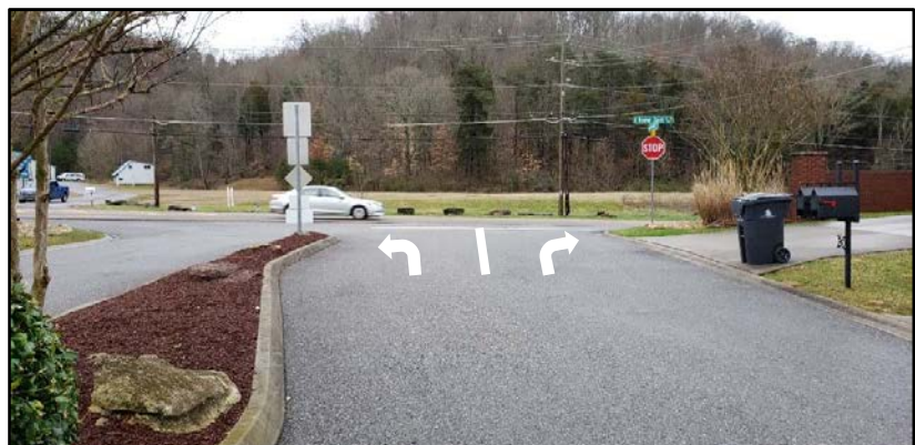
Proposed White Lane Line and Turn Arrows on Rocky Mountain High Boulevard at East Beaver Creek Drive (Looking Southeast)
