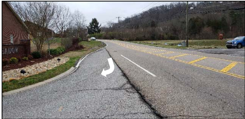
Proposed White Right Turn Arrow at Westbound Right Turn Lane on East Beaver Creek Drive (Looking Northeast)
