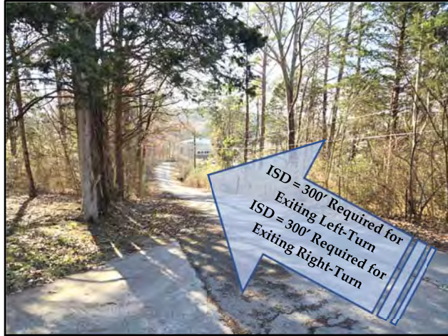
View of Sight Distance on Bradley Lake Lane at the Proposed Road "B" Entrance Location (Looking West)
