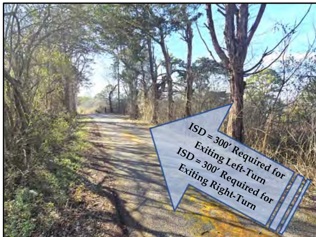
View of Sight Distance on Bradley Lake Lane at the Proposed Road "C" Entrance Location (Looking West)
