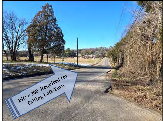
View of Sight Distance on Amherst Road at Bradley Lake Lane (Looking North)
