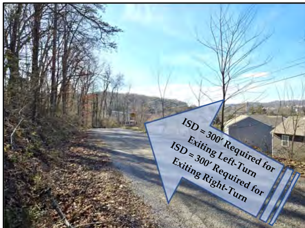
View of Sight Distance on Bradley Lake Lane at the Proposed Road "A" Entrance Location (Looking West)
