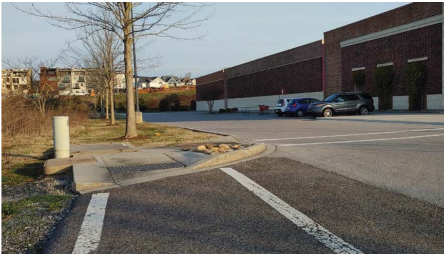
Figure 10 Line of Sight LEFT From EW Access Easement
