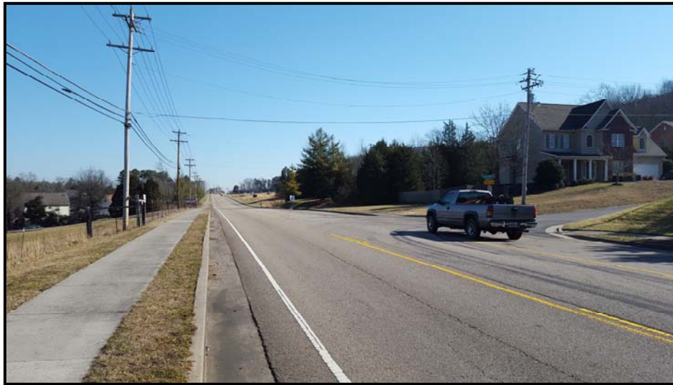
View of Hardin Valley Road at Proposed Tie-In Location (Looking Northeast)
