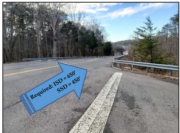
View of Sight Distance on Oak Ridge Highway at Pebblepass Road (Looking West)
