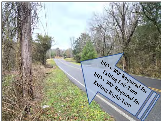
View of Sight Distance on Ellistown Road at Proposed Ellistown Road Entrance (Looking South)
