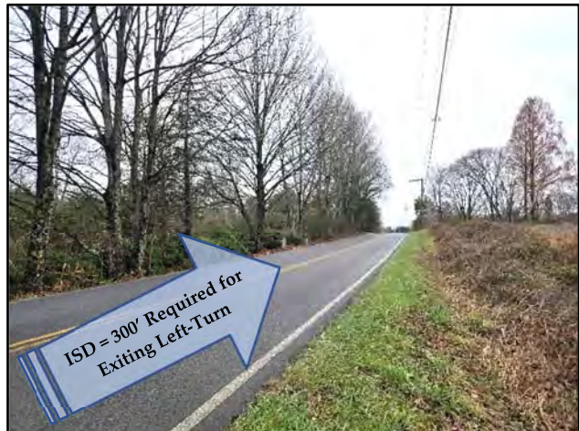
View of Sight Distance on Ellistown Road at Proposed Ellistown Road Entrance (Looking North)
