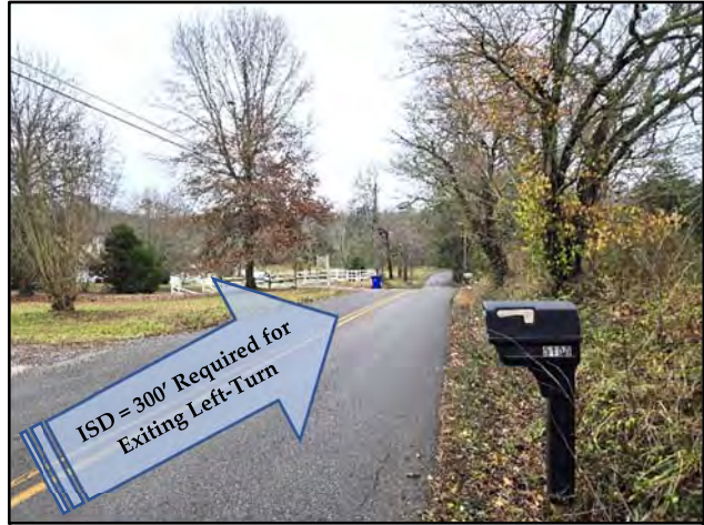
View of Sight Distance on Shipe Road at Proposed Shipe Road Entrance (Looking South)
