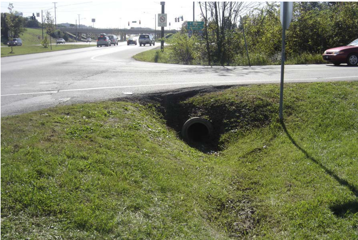
10/19/09: Looking at the northern culvert opening at Brakebill Rd.
