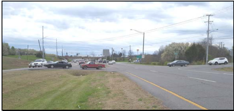
View of Median of Strawberry Plains Pike at Brakebill Road (Looking South)
