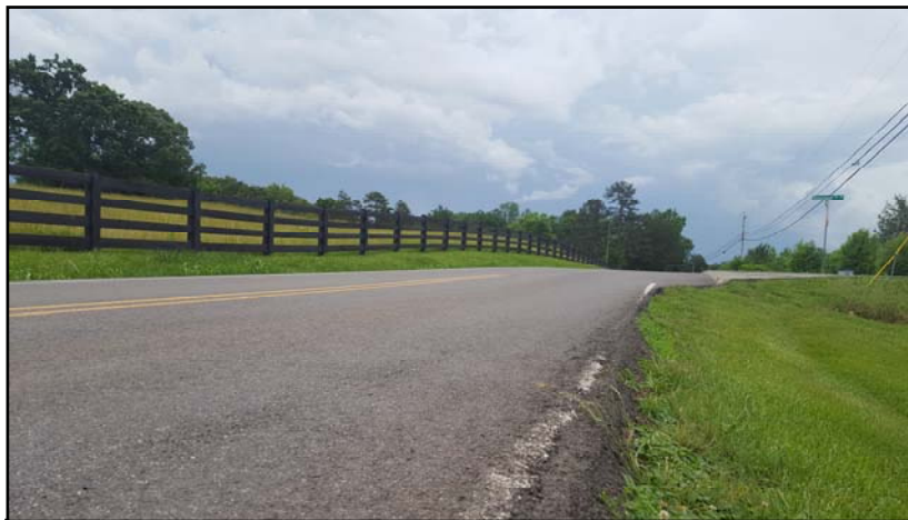
Shoulder drop-off with evidence of vehicle scraping asphalt (Looking South)
