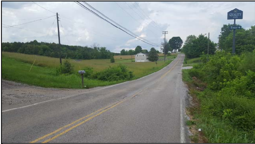
Steep road/shoulder drop-off and deteriorated pavement (Looking North)
