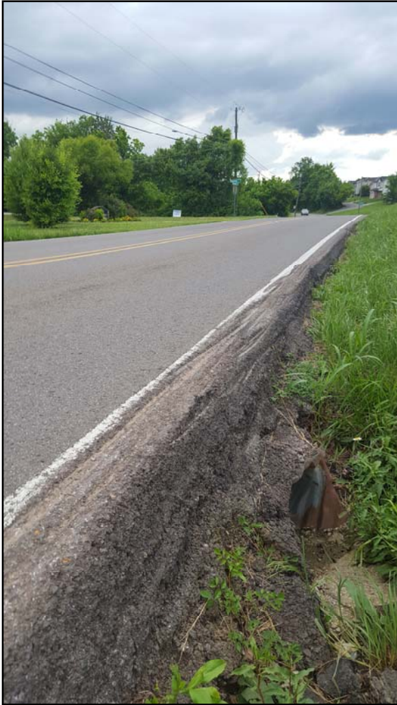
Deep shoulder drop-off into drainage ditch with evidence of vehicle scraping asphalt (Looking North)
