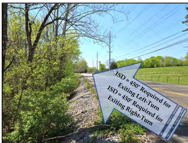
View of Sight Distance on Strawberry Plains Pike at the Proposed Entrance Location (Looking West)
