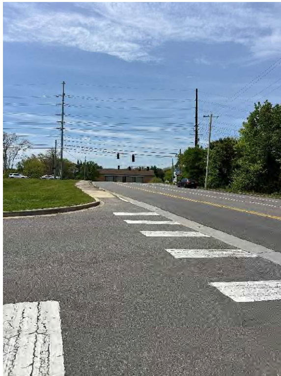
Westland Drive at Driveway – Looking Left (Westbound)
