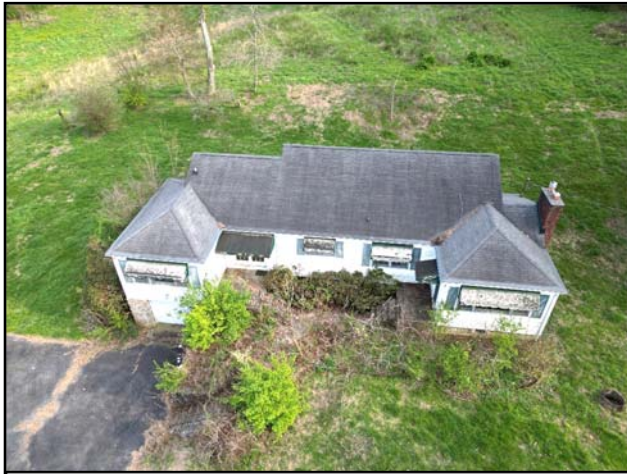
Existing Abandoned House at 11316 Hardin Valley Road
