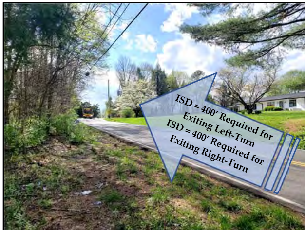
View of Sight Distance on Bob Gray Road at the Proposed Entrance Location (Looking West)
