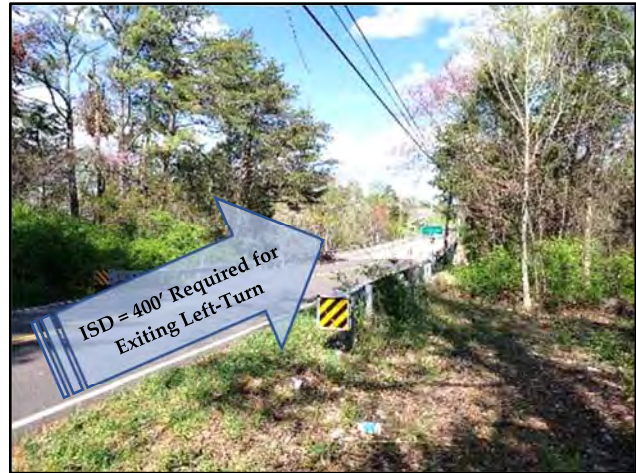
View of Sight Distance on Bob Gray Road at the Proposed Entrance Location (Looking East)
