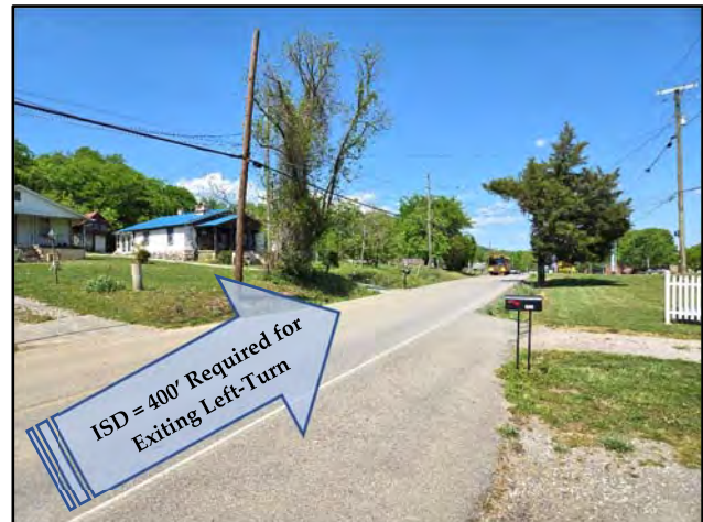
View of Sight Distance on Millertown Pike at the Proposed Entrance Location (Looking East)
