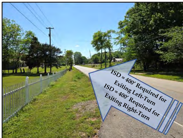
View of Sight Distance on Millertown Pike at the Proposed Entrance Location (Looking West)
