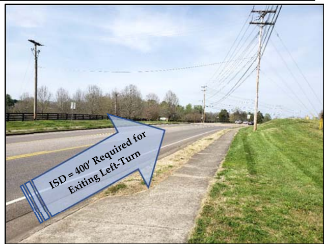
View of Sight Distance on Hardin Valley Road at the Cruz Landing Entrance Location (Looking Northeast)
