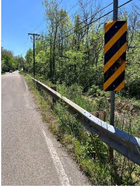
Ebenezer Road Guardrail – Southbound
