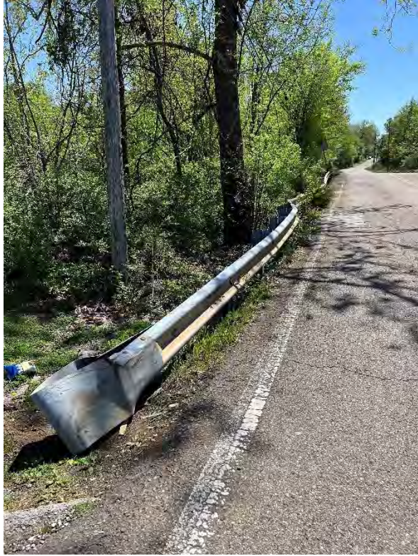
Ebenezer Road Guardrail - Northbound
