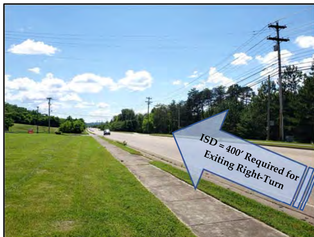
View of Sight Distance on Hardin Valley Road at the Proposed North Entrance Location (Looking West)
