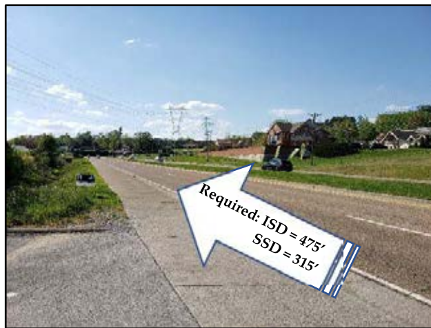
View of Sight Distance on Middlebrook Pike at Proposed Apartment Driveway (Looking West)
