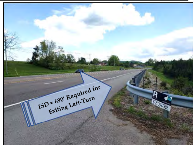
View of Sight Distance on Maynardville Pike at the Proposed Entrance (Looking South)
