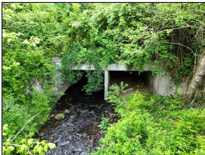
Double-Barrel Concrete Box Culvert over Mill Branch Creek at Proposed Entrance Location
