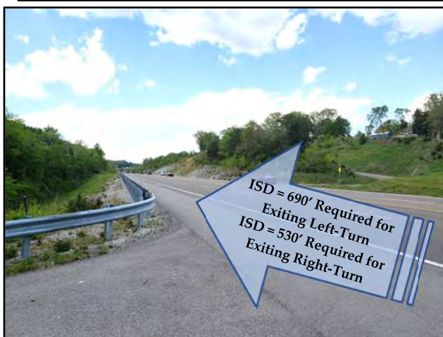
View of Sight Distance on Maynardville Pike at the Proposed Entrance (Looking North)
