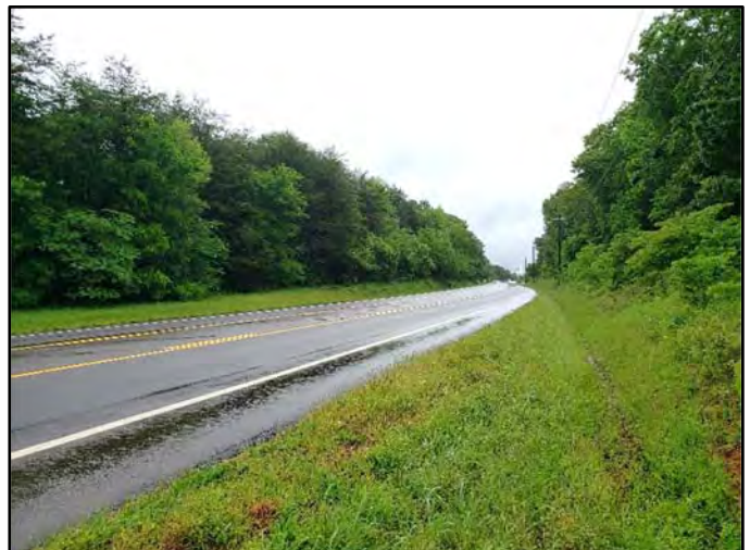
View of Sight Distance on West Governor John Sevier Highway (SR 168) at Road "B" Proposed Location (Looking East)
