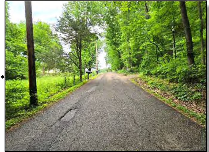
View of Carter Mill Drive (Looking Northeast)
