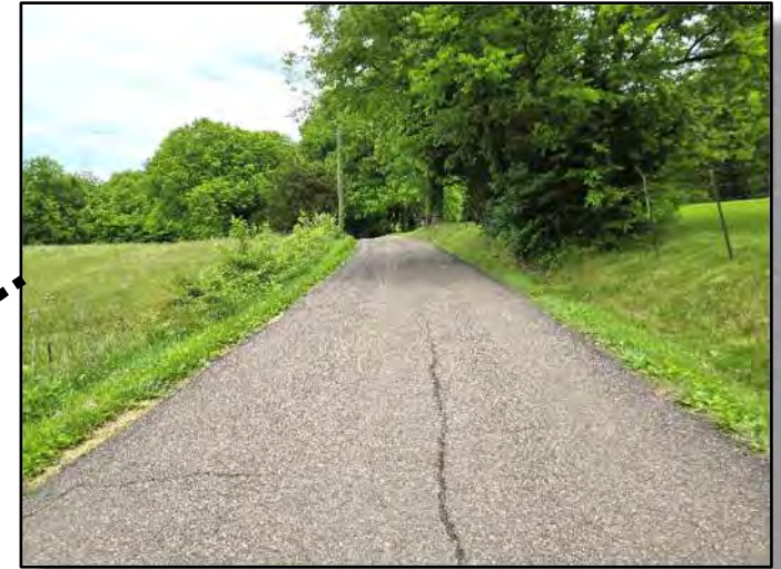
View of Carter Mill Drive (Looking Northeast)
