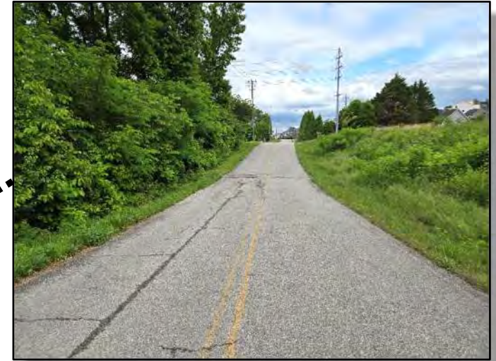
View of Carter Mill Drive (Looking Northeast)
