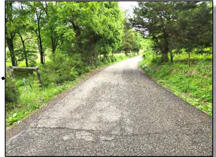
View of Carter Mill Drive (Looking Northeast)
