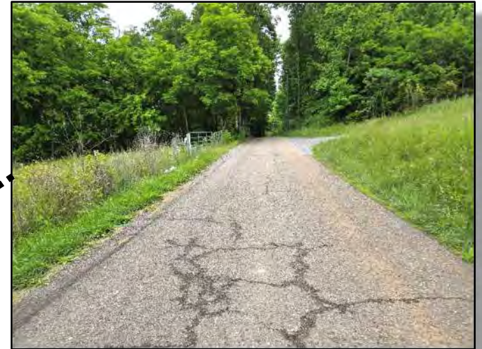
View of Carter Mill Drive (Looking Northeast)
