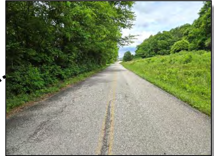
View of Carter Mill Drive (Looking Northeast)
