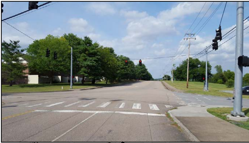
View of Millstone Lane at George Williams Road (Looking Northeast)
