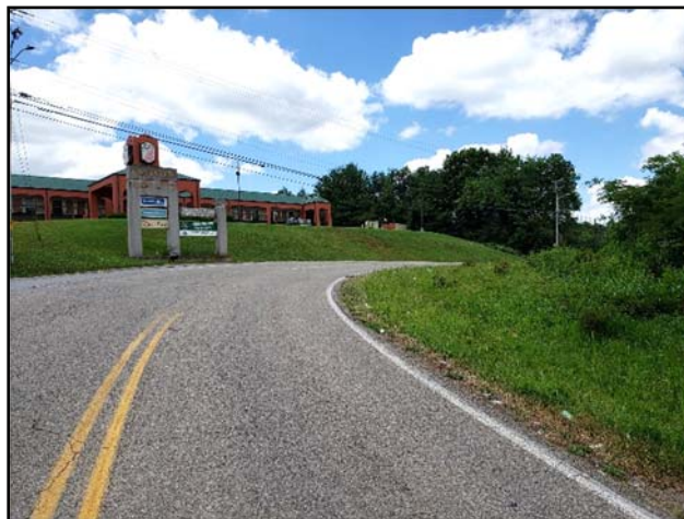
Roadside vegetation obscures sight distance for turning vehicles at Crosswood Boulevard and Brakebill Road (Looking Northwest)
