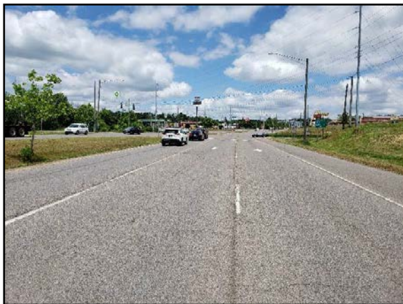
Single Left-Turn on Strawberry Plains Pike at Interstate 40 On/Off-Ramps (Looking North)
