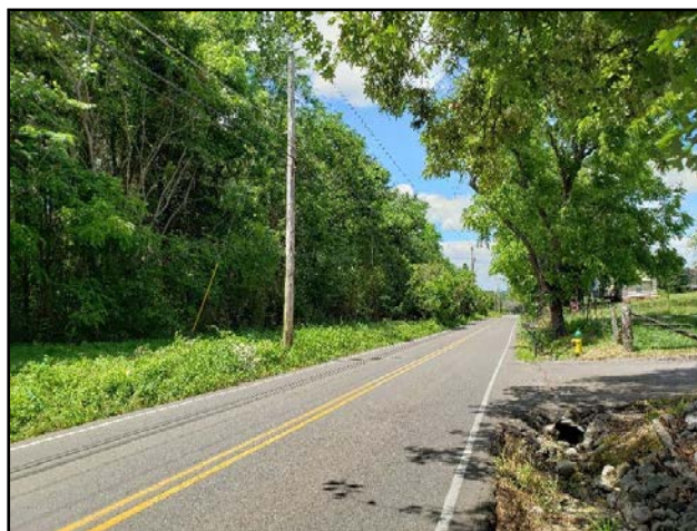
Large trees and utility poles adjacent to the roadway near 512 Brakebill Road with shoulder drop-off into the drainage ditch (Looking North)
