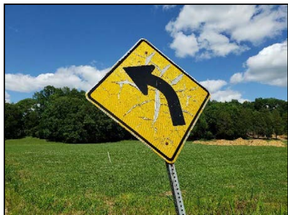
Deteriorated Curve Sign for NB Traffic on Brakebill Road near Kilbridge Drive
