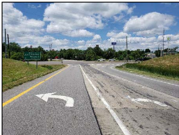
Double Left-Turn on Interstate 40 Off-Ramp at Strawberry Plains Pike (Looking West)
