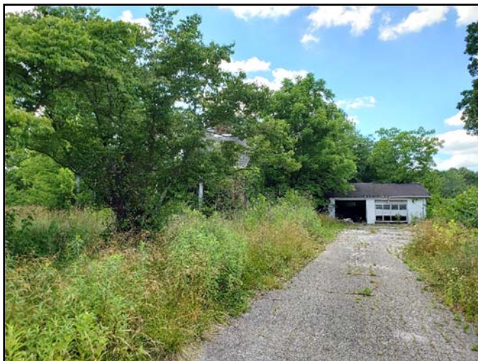
Abandoned Residence on Site Property
