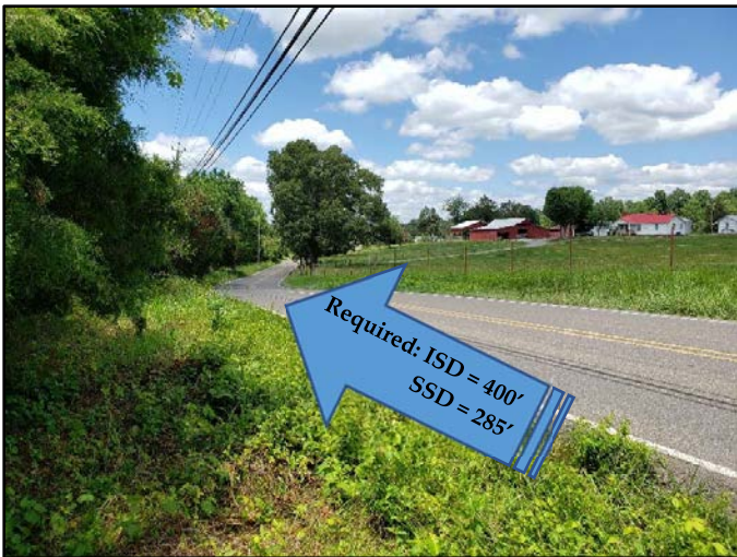
View of Sight Distance on Brakebill Road at Proposed Road "A" Intersection (Looking North from Road "A" Location)
